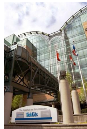
Facilities Director Ron Lowe’s annual energy savings target is $2 million at Toronto’s Hospital for Sick Children
